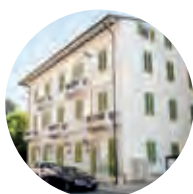
Santa Rita Hospital Montecatini Terme (PT)
